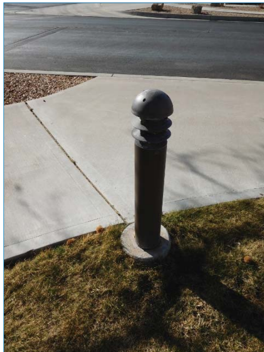
Typical bollard light fixture
