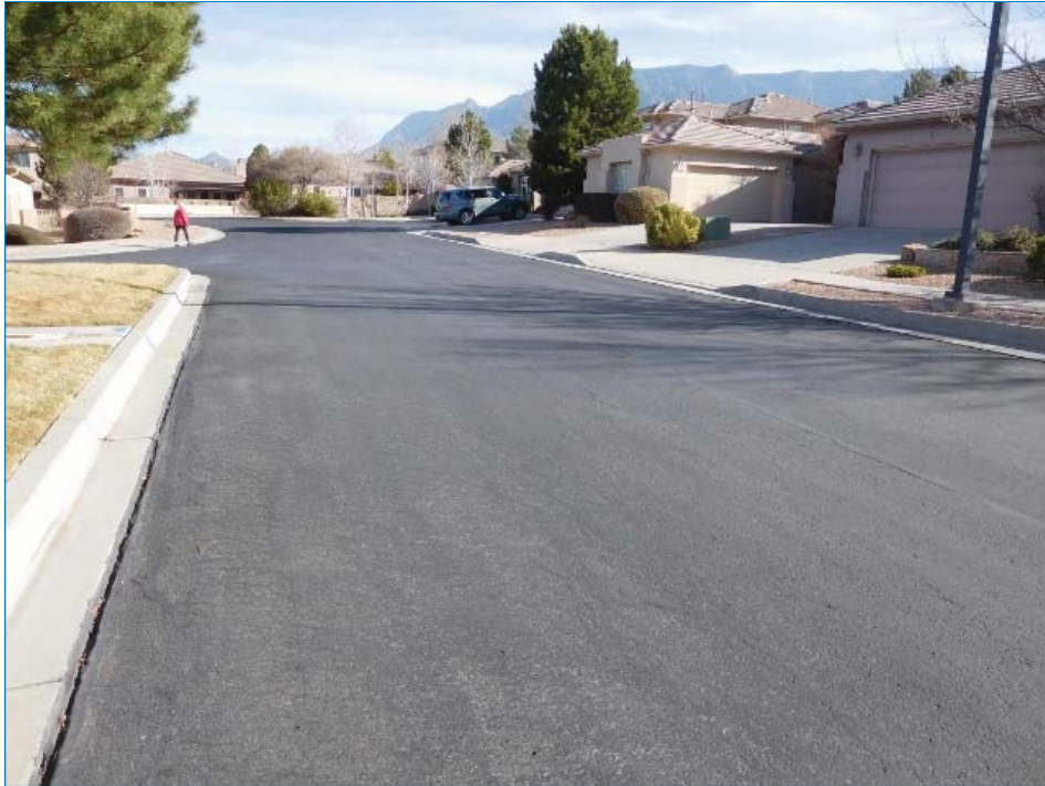
Typical street asphalt
