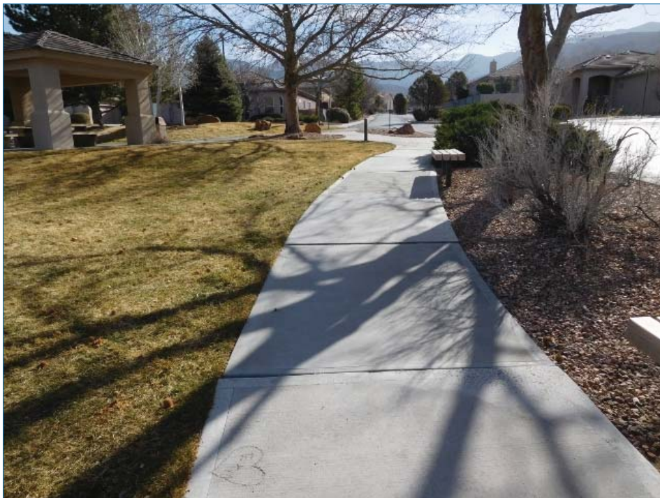
Typical concrete walkway
