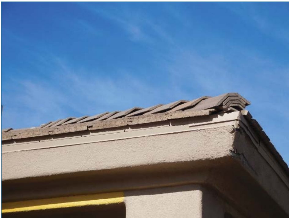
Typical concrete tile roofing
